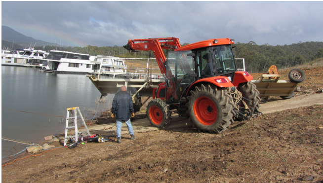
Garry & Ronnie carrying out marina repairs in May.
