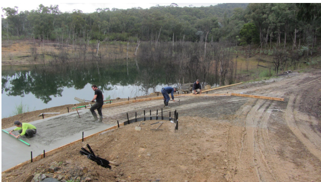
Onsie & Twosie labouring for the concreters!
