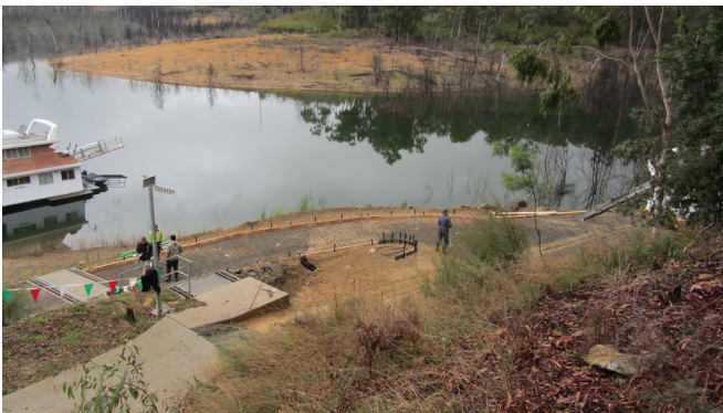
Concreting preparations at A Marina
