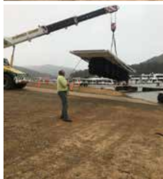
From factory to the water. The new marina sections being fabricated, transported, assembled on site, craned to the lake, and placed into B&D marinas. All in a days work.....
